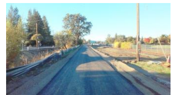
Views of current construction between Yountville and Napa
